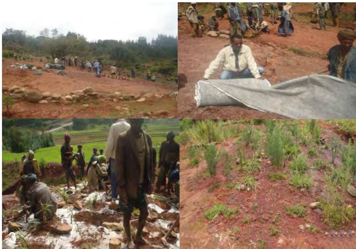
Figure 21. Watershed management through the Application of biodegradable geotextile for the rehabilitation of degraded land in Lake Tana catchment (Source: Zerihun, 2016)
